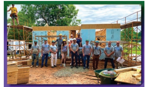
A Habitat house under construction
